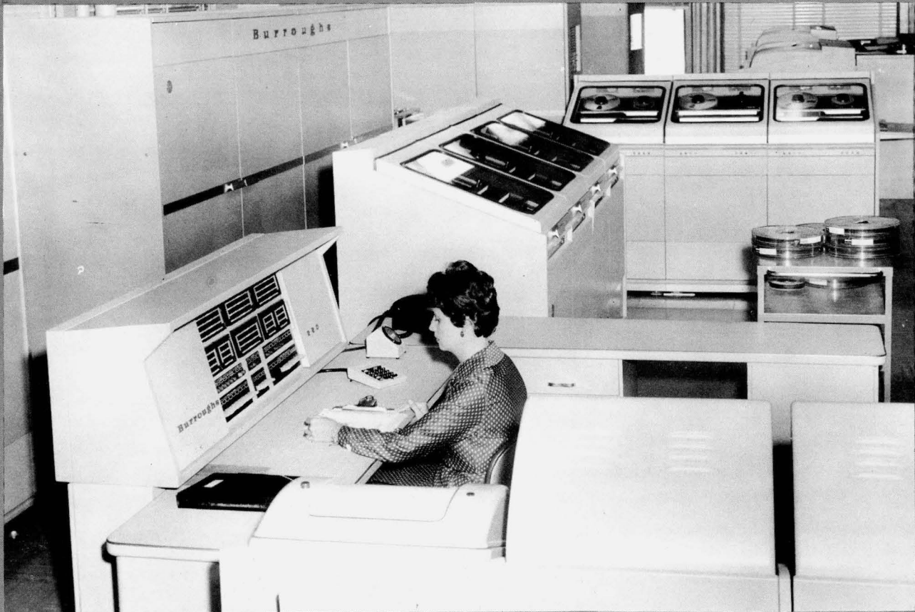
-- Console and tape units of one of the two Burroughs 220 electronic computers installed as part of the fully automatic electronic bank bookkeeping system at the First Pennsylvania Banking and Trust Company, Philadelphia. Information recorded on magnetic tape by the B 301 Magnetic Document Processing system provides input to up-date customer account records which in turn are used to prepare customer statements. Virtually every banking operation can be carried out using this system. --
