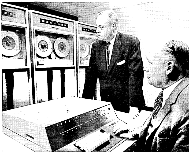
AN/UYK-1 digital computer -- Ramo-Wooldridge, division of Thompson-Ramo-Wooldridge Inc., Canoga Park, Calif. This multiple-purpose digital computer is claimed to have achieved a degree of versatility and user convenience not ordinarily possible in an inexpensive computer by using "stored logic" techniques. This permits the user to select a word length, order structure, and instruction repertoire especially suited to the problem at hand. These normally "wired in" characteristics are specified by data stored in the computer's memory and may be changed during the normal loading procedures without hardware modifications.
