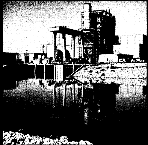
At San Antonio's City Public Service Board... automatic turbine startup... monitoring, alarming and display functions... and direct digital control on selected control loops.
