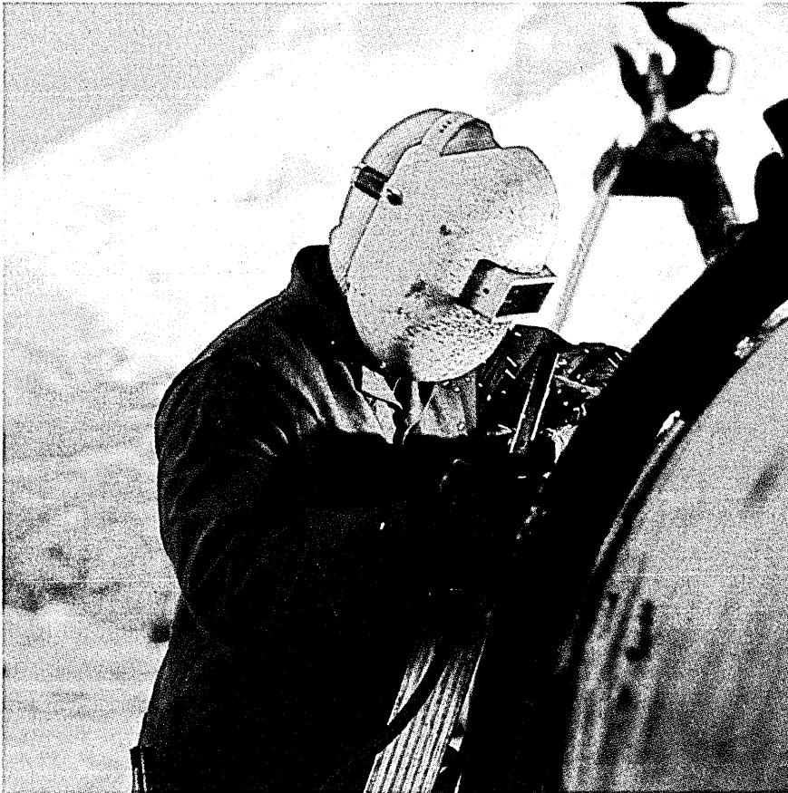
A pipe casing is welded on the Alaska pipeline. To help manage the $7 billion project, the Alyeska Pipeline Service Company is using an IBM System/370 Model 145.
