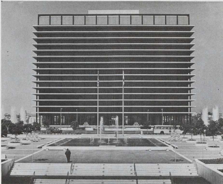
Solid state affords precise environmental control throughout large complexes like Los Angeles' Water and Power Building. Page 17
