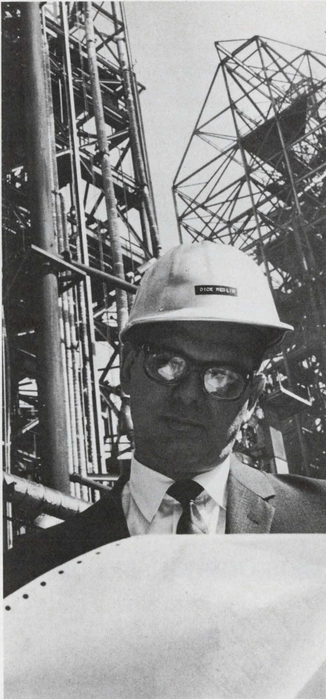
Direct digital control (DDC) is taking over in many big plants like this oil refinery. Page 17
