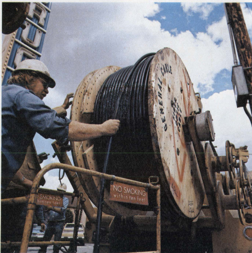
Fiber-optics cable for a 5.6-mile telephone system in California is pulled through an underground conduit. The 1.544-Mbit/s system, developed by General Telephone and Electronics, uses cables by General Cable Corp.
