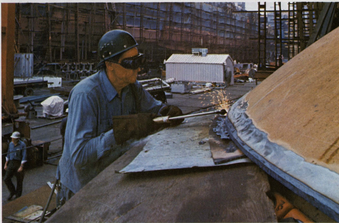
This welder at Ingalls Shipbuilding, has access to an IBM computer to verify that his construction drawings are up to date. Workers and engineers throughout the huge shipyard access a wide range of computer applications through nearby terminals.
