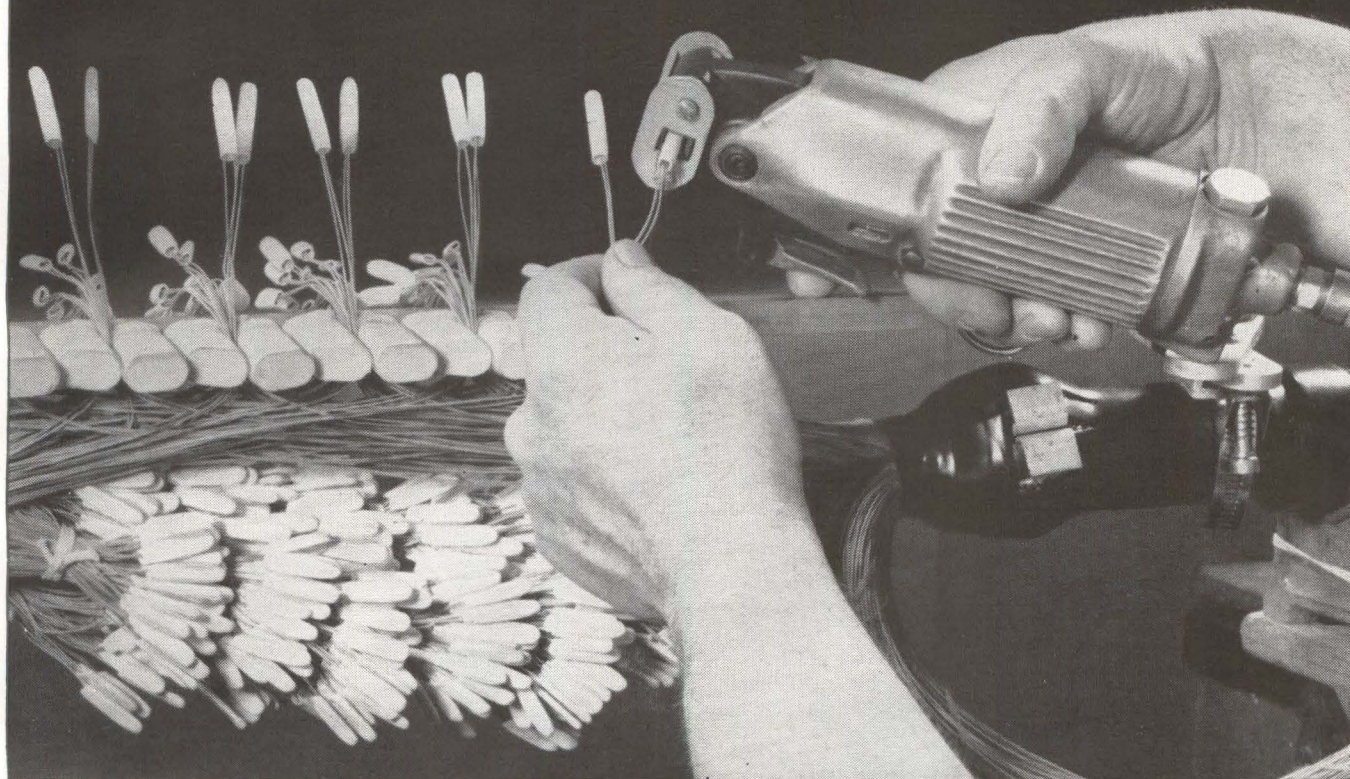
Telephone craftsman uses special pneumatic tool to flatten connector onto insulated wires. Metal tangs pierce insulation and produce a splice that is equivalent to a soldered joint.
