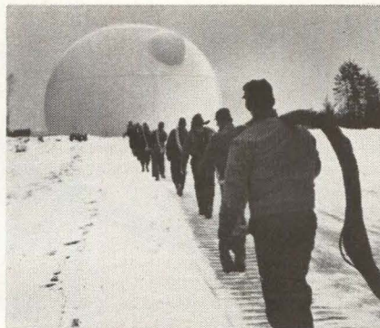
Antenna at the Andover tracking station was erected this winter. Cable is shown being carried during construction.
