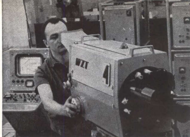
STUDIO TV CAMERA from Poland can be remotely controlled
