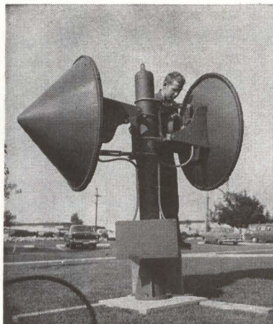
BISTATIC doppler radar installed by Sylvania at Nike Hercules missile base detects person stepping inside electromagnetic field
