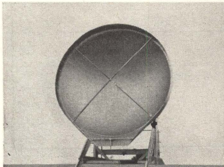
■ 20 meter diameter antenna for satellite communication
