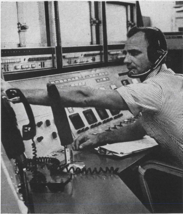
When a Minuteman missile launched from Cape Kennedy reaches an altitude of 60,000 feet, RCA engineer Sam Lynch picks it up on Mistram 2 at Eleuthera. The entire Mistram 2 complex is operated at this console.
