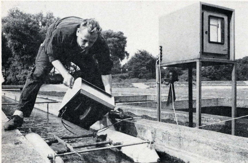
Immersed. Oil contamination in conduit of water-treatment plants is detected by drop in conductivity across electrode pairs mounted on wheel that spins with its rim dipped.
