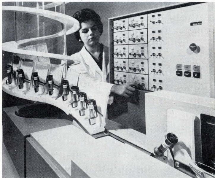
**Automated lab.** Experimental equipment demonstrates a possible scheme for rapid analysis of blood samples. Specimen is poured into a funnel and analyzed by conventional laboratory instruments. Signals from the instruments are converted by a control unit into computer-readable form, and the computer then calculates test results and prepares a report.
