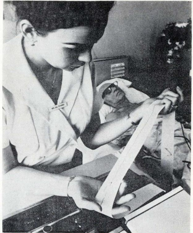
**Bedside consultant.** Portable electrocardiograph sends EKG signals over a telephone line to a remote computer for analysis. The signals are also recorded in the conventional manner for immediate analysis by a doctor.
