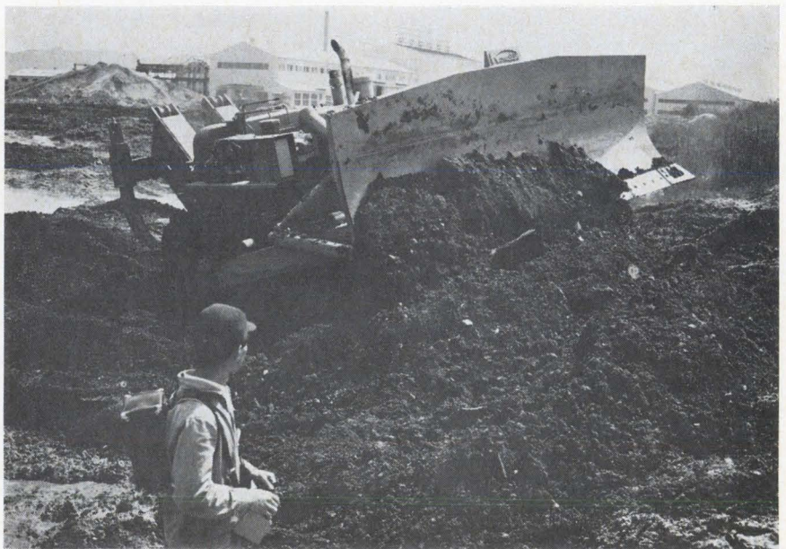
Sidelined. Unskilled operator fiddling with joysticks can put bulldozer through its paces like a veteran cat skinner.
