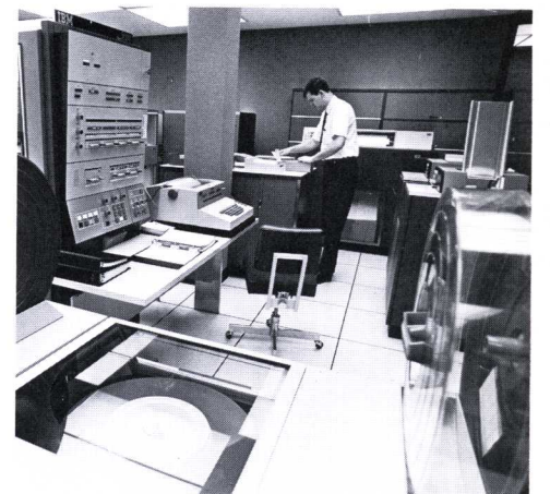
Portion of computer room.
